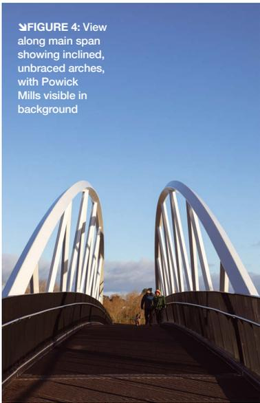
FIGURE 4: View along main span showing inclined, unbraced arches, with Powick Mills visible in background
