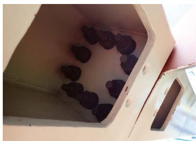
**FIGURE 16:** Hidden bolted splice connection within edge beams (cover plates omitted)
